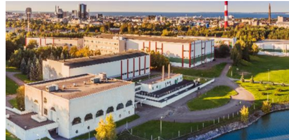
Ülemiste Water Treatment Plant
